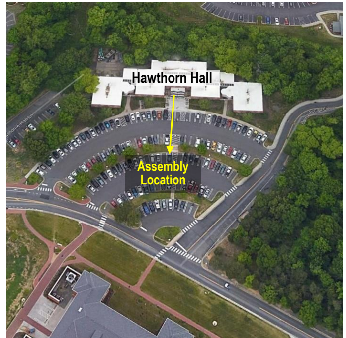
Hawthorn Hall - Site Photo
